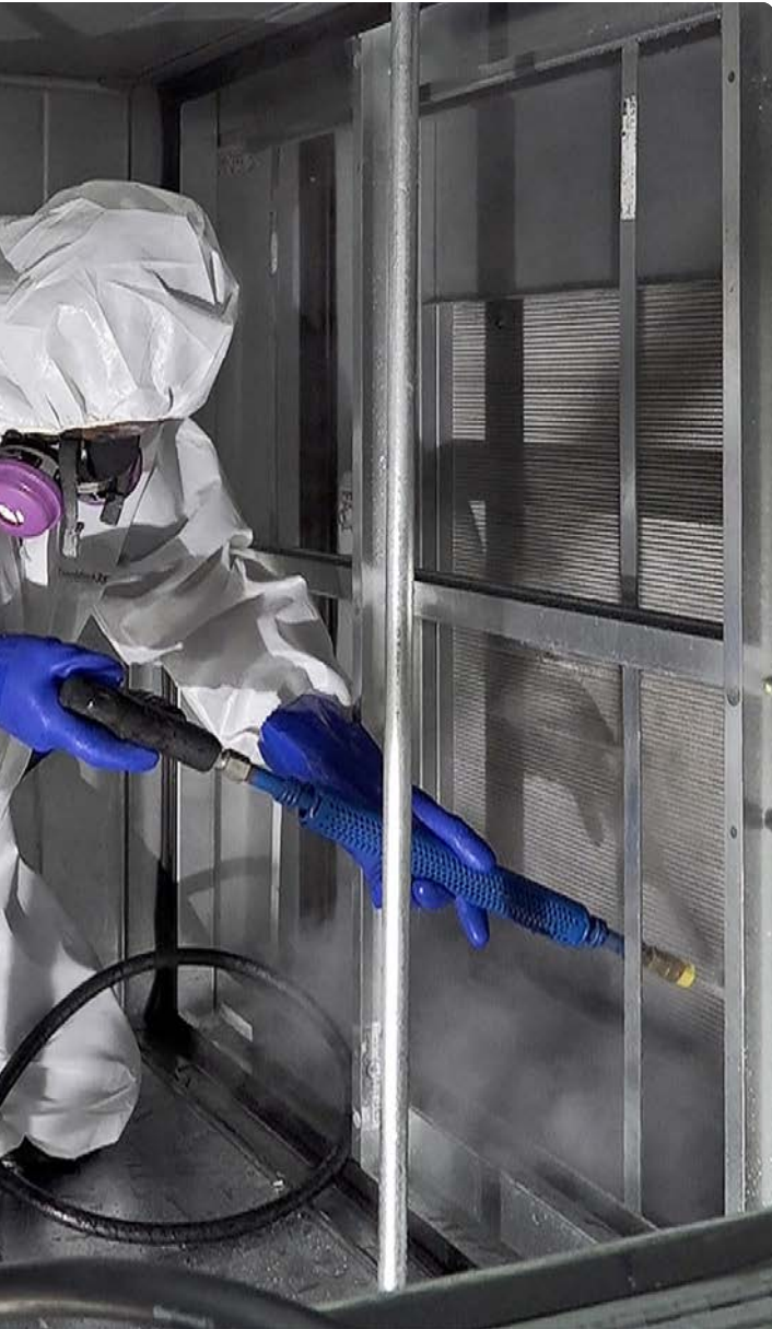
Pure Air helps facilities disinfect their HVAC systems with high temperature steam to restore airflow and energy efficiency while also improving air quality.
